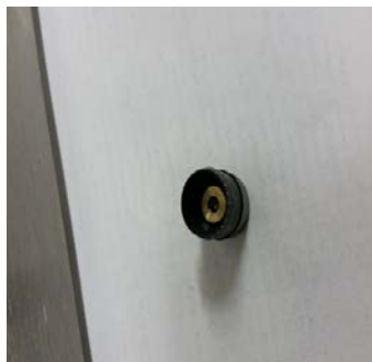
Figure H.1: Detached Flow Adjust Valve
